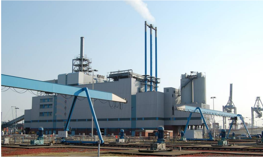
VERA – sludge incineration plant
