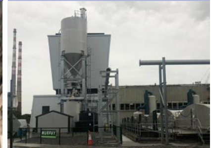
View of P-Fix Building and MgO Storage Facility
