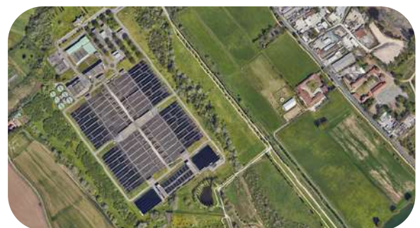
Areas identified in agreement with MM technicians and the Municipality of Milan for the construction of phytoremediation systems
