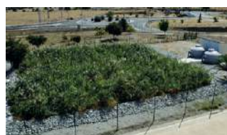
Artificial wetland with hydrolytic anaerobic digester to remove nitrogen
