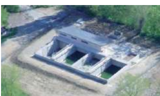
Sequential batch reactor
